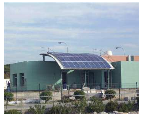
6.12 kW on a curved roof in the Information Point for the La Breña y Marismas Natural Park in Barbate (Cádiz)
