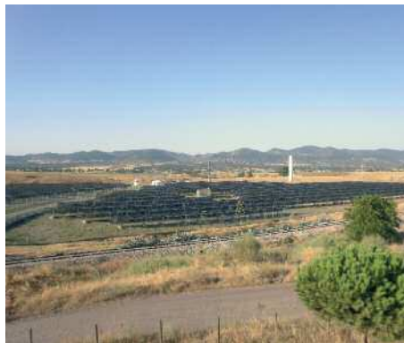
1.7 MW overground in a permanent structure in Peñarroyo-Pueblonuevo (Córdoba)
